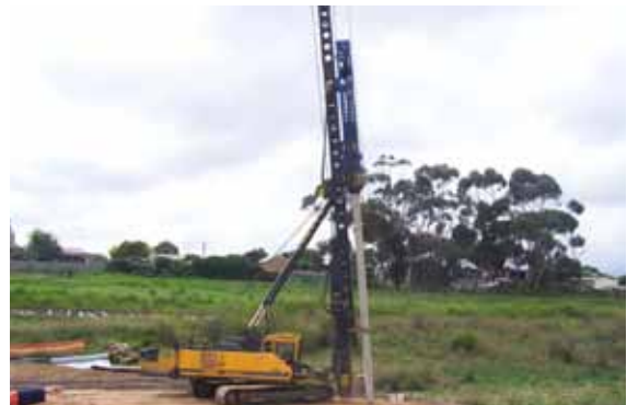
January 2011 commenced piling works
