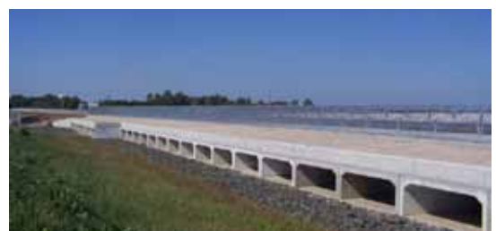
Completed western approach
