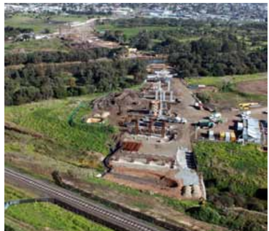
July 2011 aerial photo of progress
