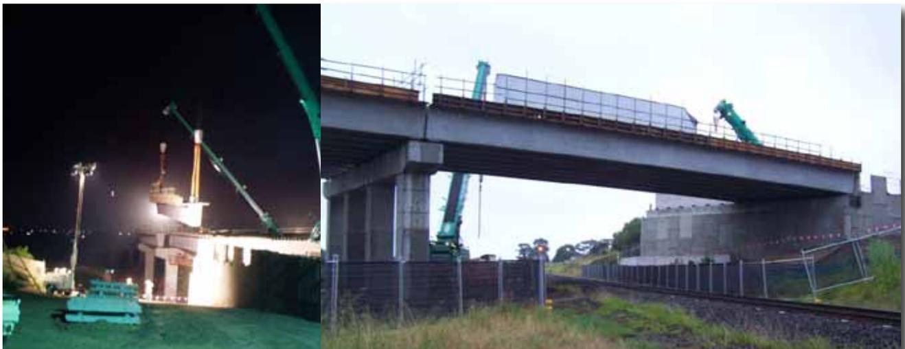
*Installing the final span over the rail line, 25-28 November 2011*
